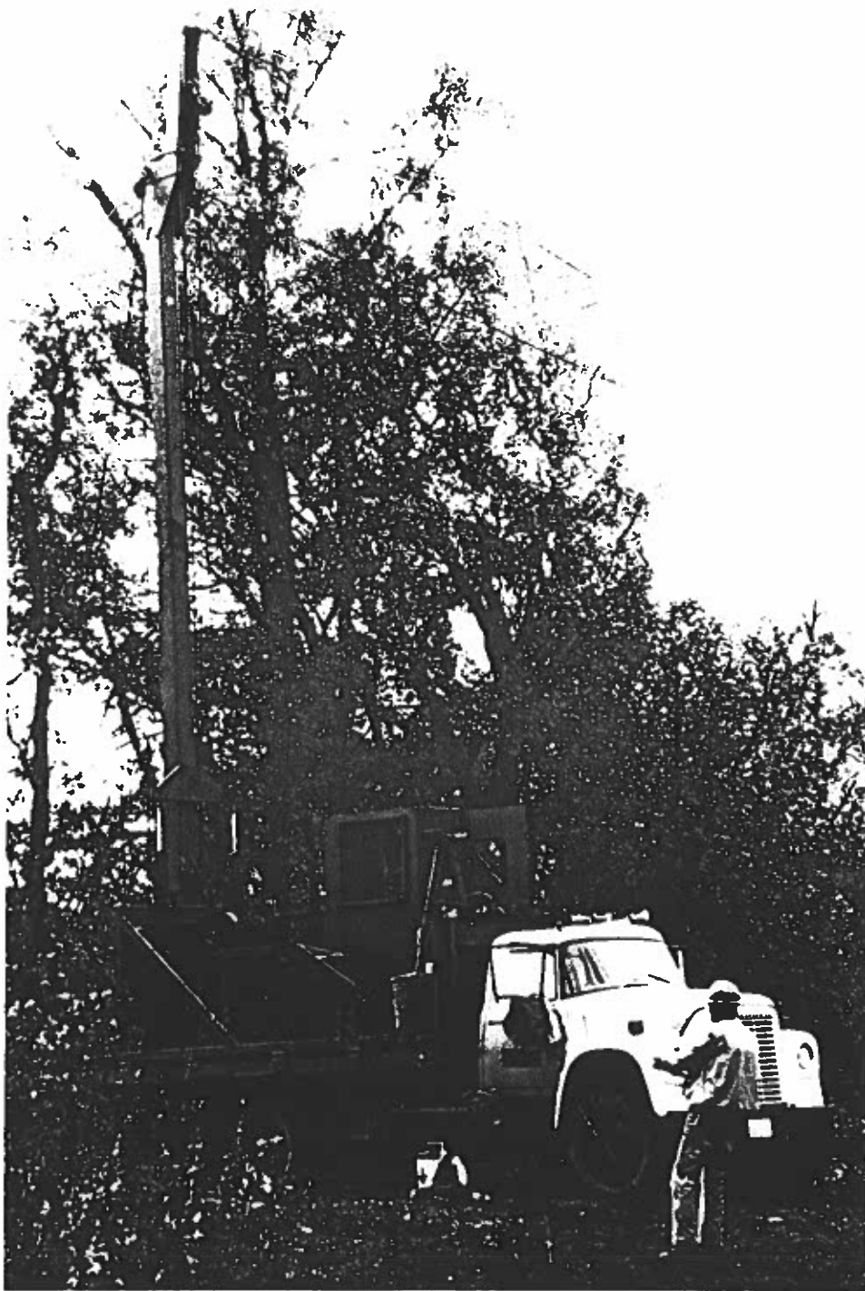
Figure 2. The Clearwater double-drum skyline cable yarder used in this study.
